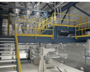
Greenfield & New Equipment
